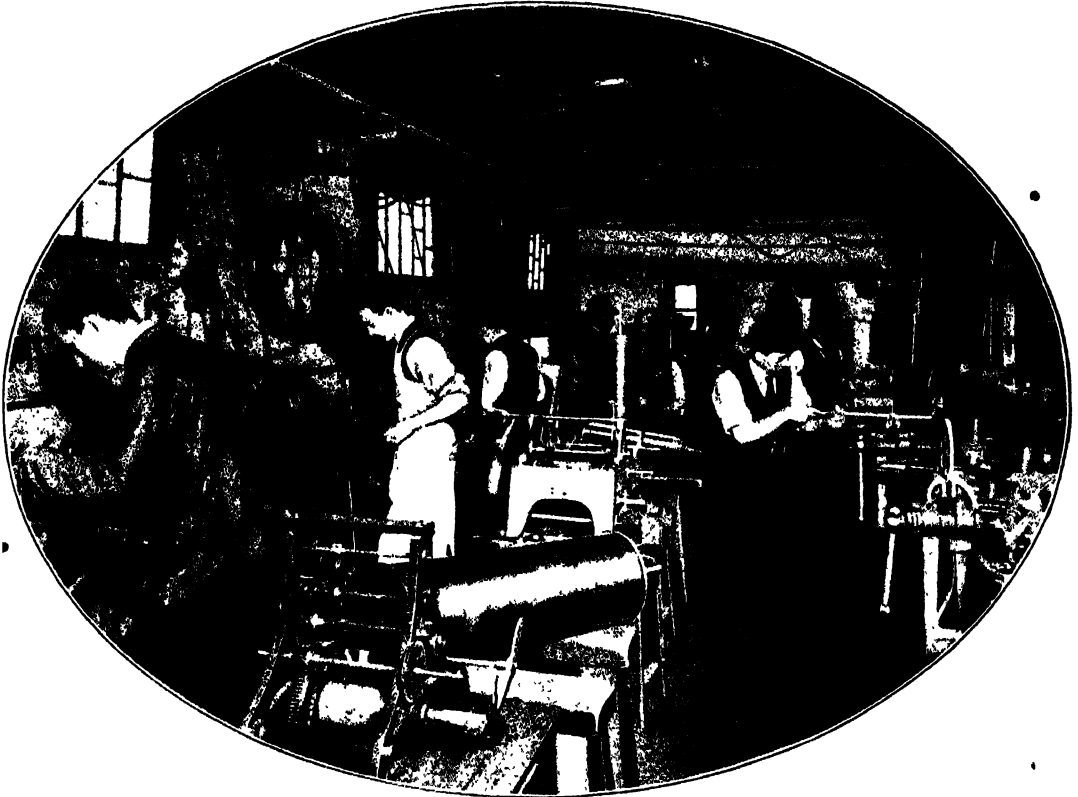
CLOCK-MAKING : PUTTING THE MOVEMENTS TOGETHER.
